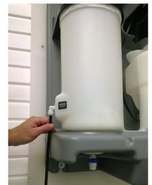
5. Install the fitting (thread sealant not included) you will need to connect to; a feed pump (push-in elbow fitting) or HydroDose (barb fitting) on the side port labeled "Chemical Outlet" and connect your tubing to the fitting. **IMPORTANT: Ball valve at the bottom of the unit is for a drain only. DO NOT draw chemical from this port.**
